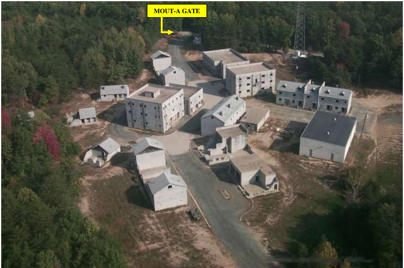
MOUT FROM NORTHWEST CORNER LOOKING SOUTHEAST
