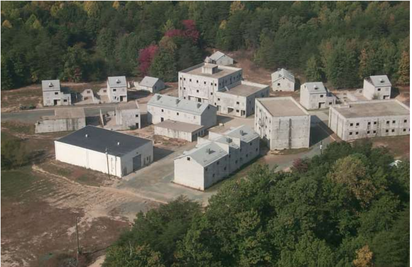
MOUT FROM NORTHWEST CORNER LOOKING SOUTHWEST
